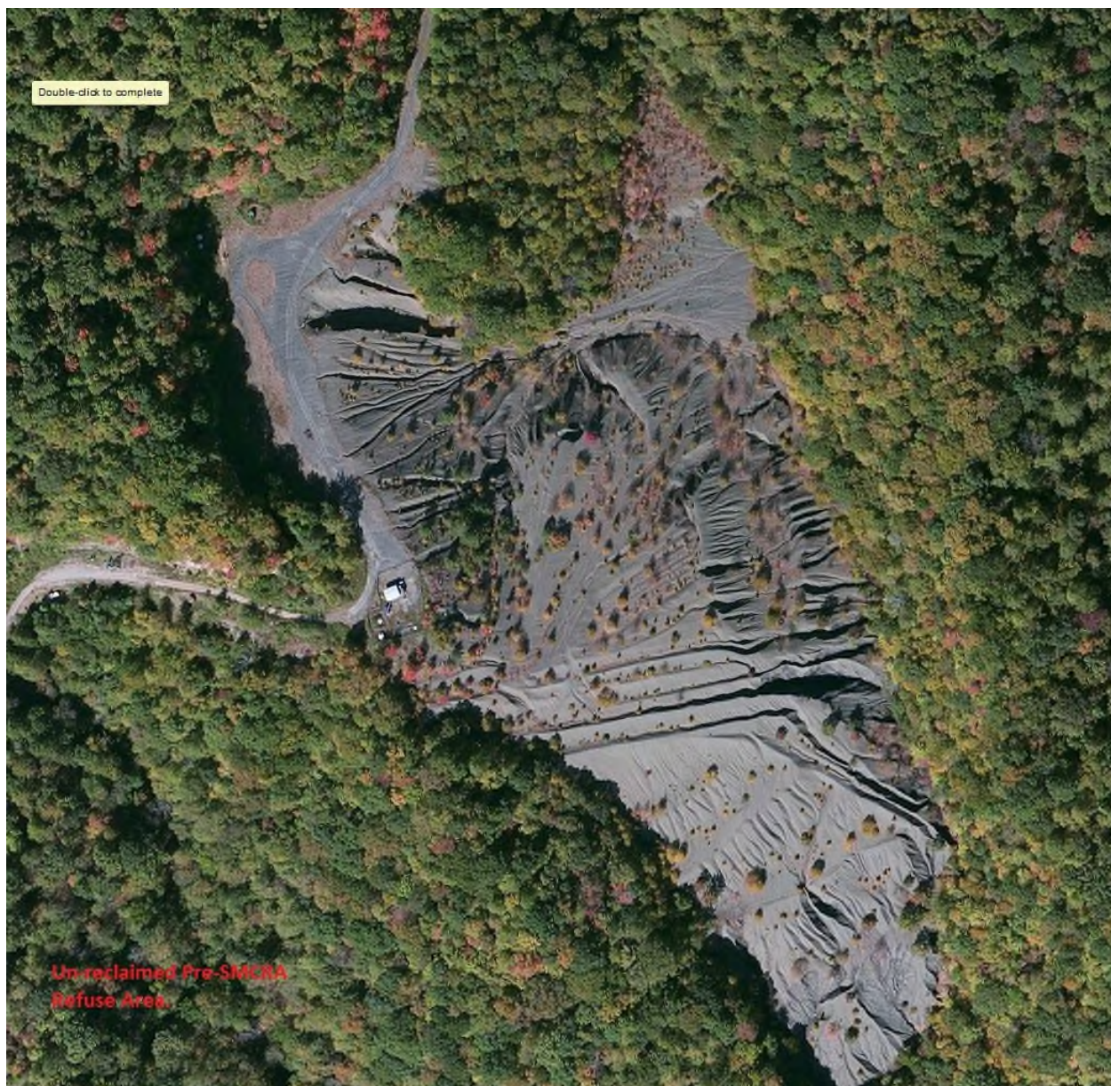
Unreclaimed Pre-SMCRA Refuse Area immediately to the East of the Crany Impoundment.
